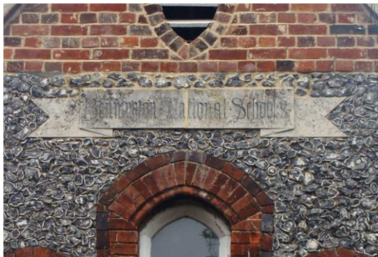
Pictures 16-17. Bennington School Parts of the building are visually most worthy of retention. Note spelling of Bennington (with double n) in centrally located stone detail.
