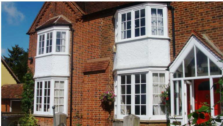
Picture 13. Beech House although some modern additions detract, the historic parts of the building are worthy of retention.
