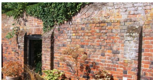
Picture 23. Brick wall Bury Lodge Farm worthy of retention.
